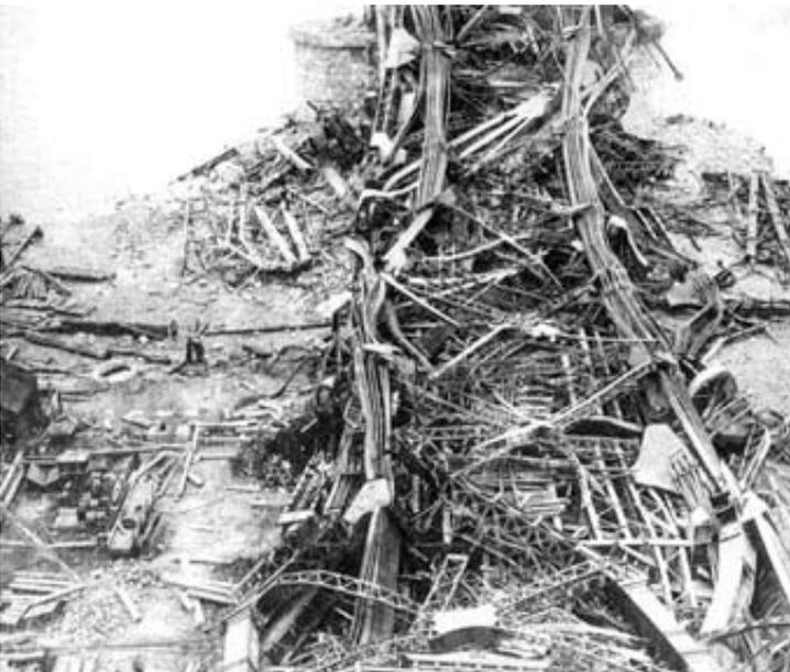
The twisted steel wreckage of the Quebec Bridge after its collapse August 29, 1907 (courtesy National Archives of Canada).
